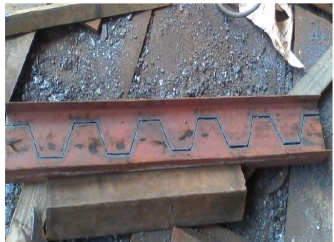
Fig-5: Gas cutting done through the markings for hexagonal shaped openings
