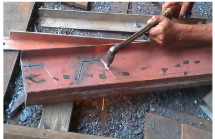
Fig-4: Gas cutting of hexagonal shaped openings
