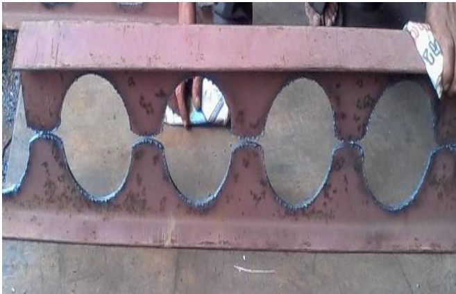
Fig-7: Gas cutting done through the markings for circular shaped openings
