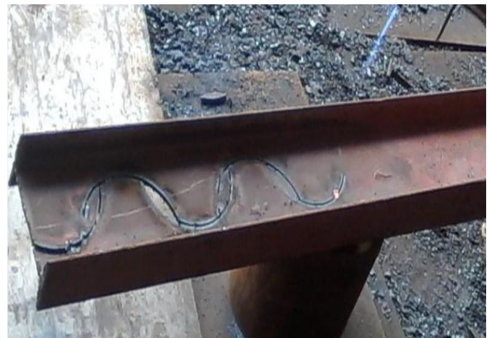
Fig-6: Gas cutting of circular shaped openings
