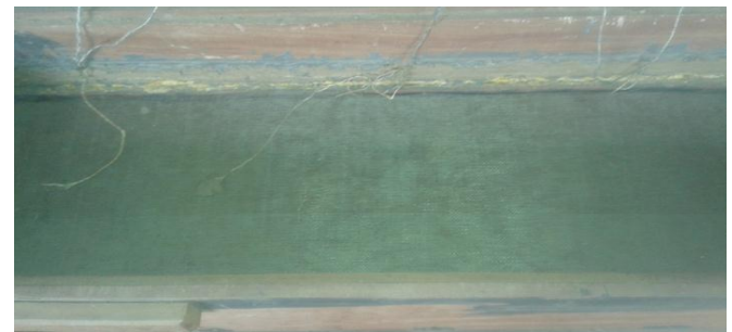
Fig.4: Duct packed with wire mesh
