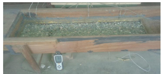
Fig.6: Duct packed with gravels
