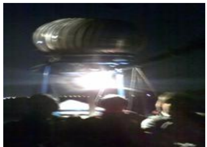
Figure 2. Wind Turbine Ventilator Generating Electricity
