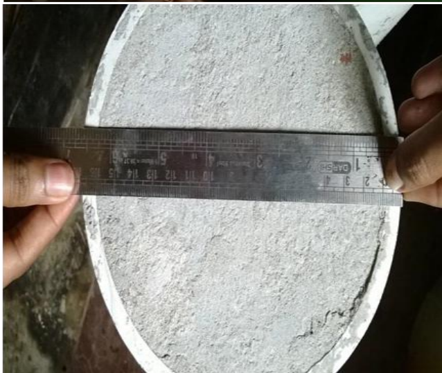
Plate(5) Failure of PVC Tube
