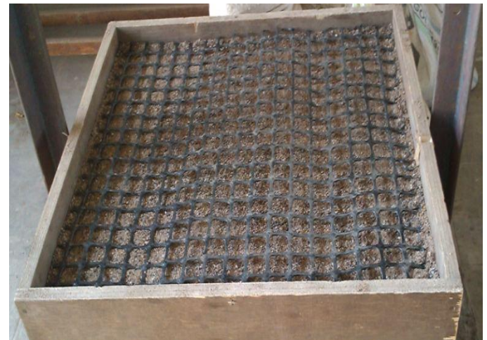
Fig 3 Placing of geogrid at 3.3cm from the base of the footing
