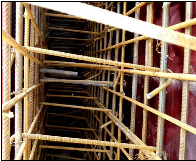
Fig -2: Moulds placed upto mid-depth of wall
