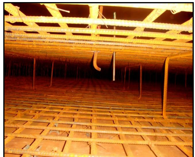
Fig -2: Moulds placed upto mid-depth of slab
