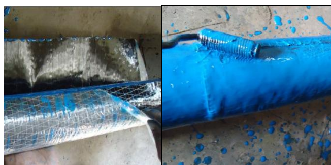
Fig-5: CFRP Wrapping (CF-3H).
