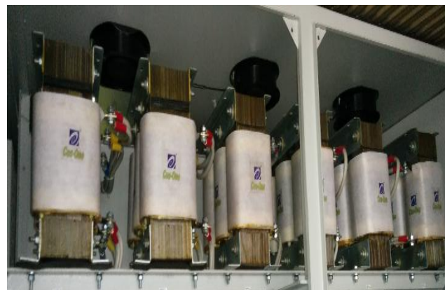
Fig. 14 Reactors installed in panel
