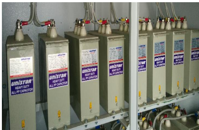
Fig. 12 Capacitors installed in panel
