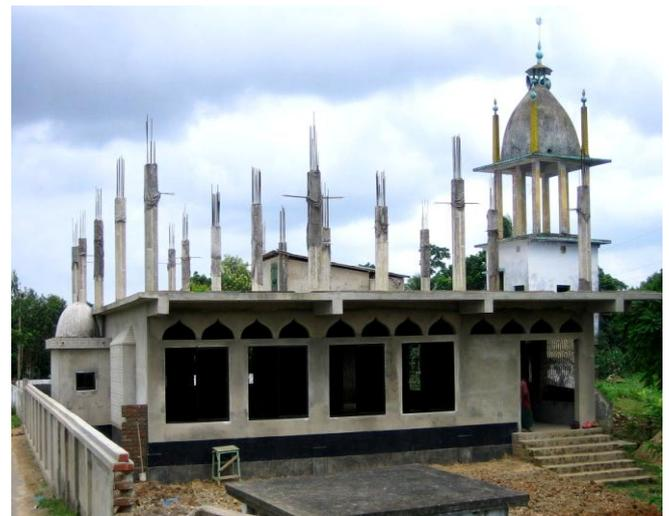
Fig: 17: Vertical extension with permanent structures.
