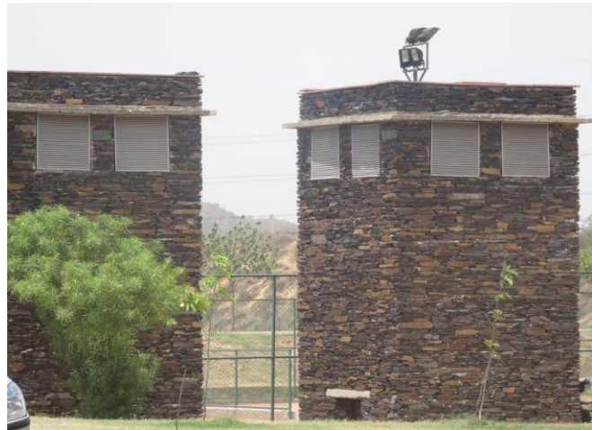
Fig -19: Towers to capture dry air from surrounding
