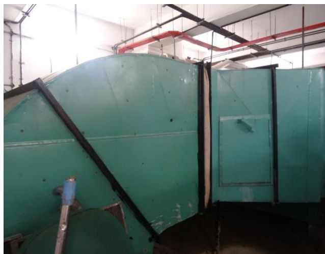
Fig -20: Air handling unit
