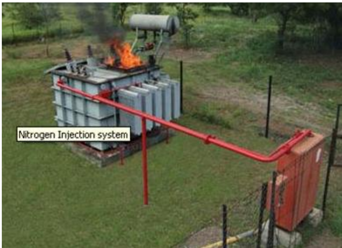
Fig -2: Transformer Installation caught by Fire
