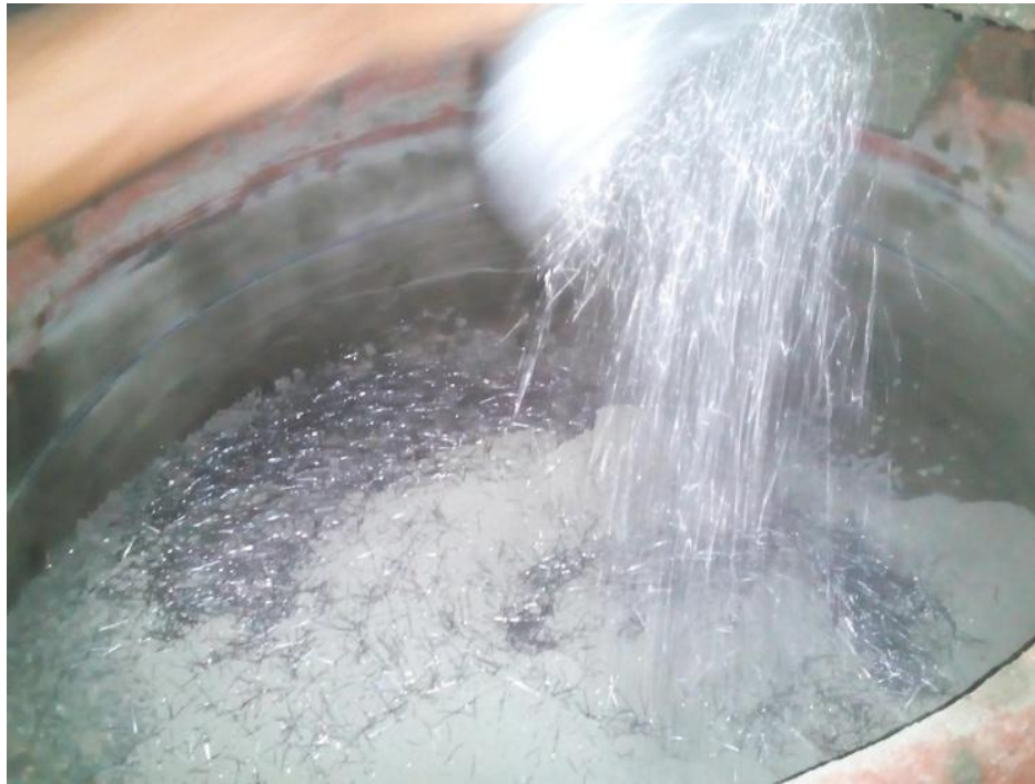
Fig -1: Addition of steel fibers in mix
