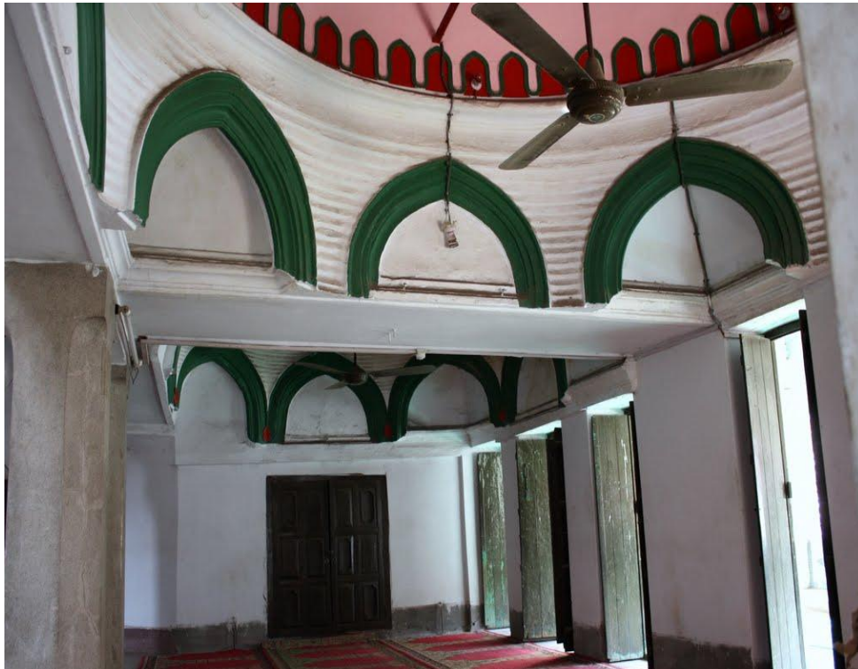
Fig:5.1.4: View of double dome from interior
