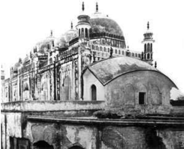
Fig: 1. Do- chala ( double roof) structure of Pre-Mughal tomb
