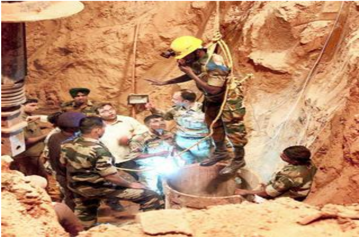
Fig -2: Army members working for the bore well rescue
