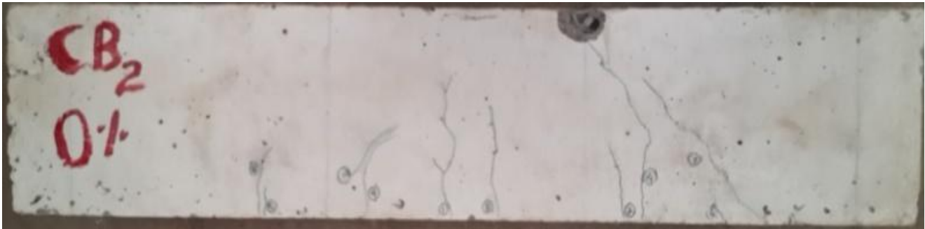
Plate 5.Failure pattern of conventional concrete beam CB
