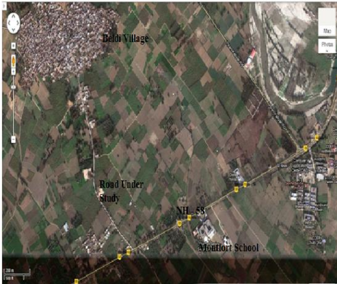
Fig -2: Shows the google map image of road under study. The road stretch is almost straight and does not required any cross drainage work.
