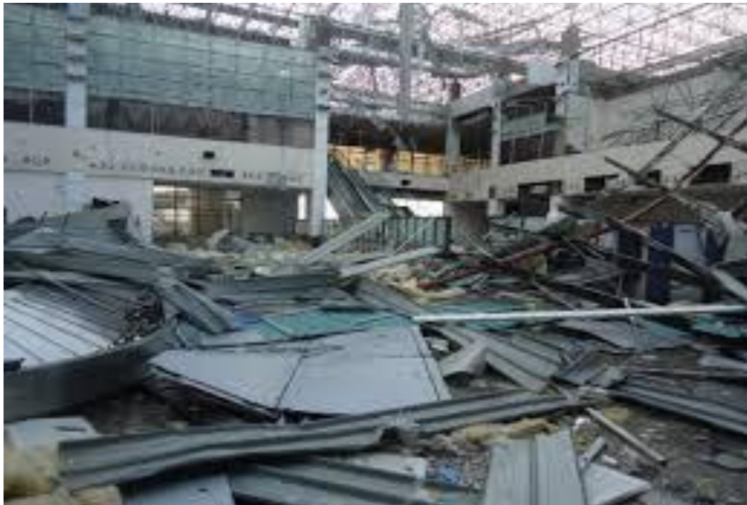
Images of Structural and non structural failures during the Hudhud cyclone in Vizag
