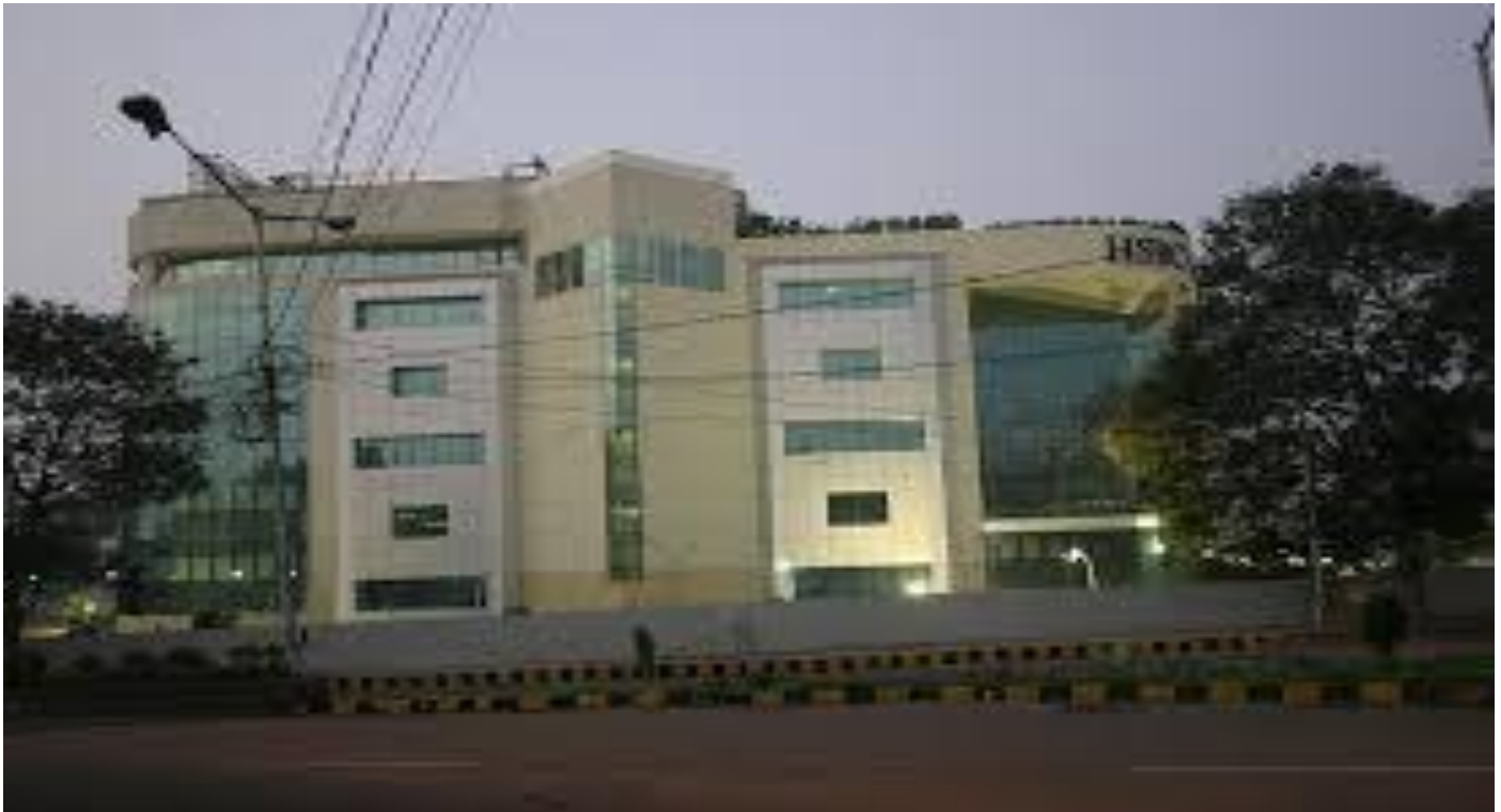
HSBC Building in Visakhapatnam, the structure served without any damage
