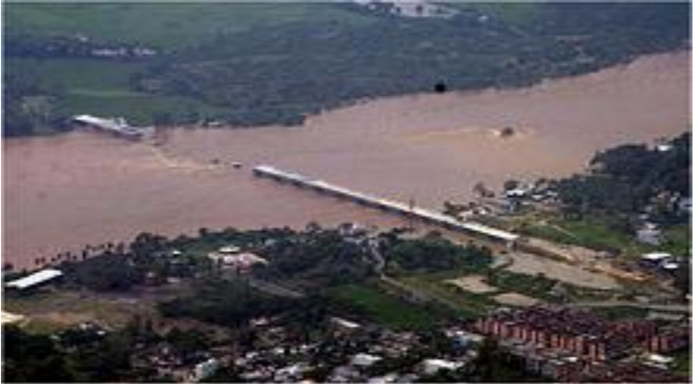
A Blown away bridge near Visakhapatnam:
