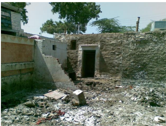
Photo 11 : Building with mud walls
