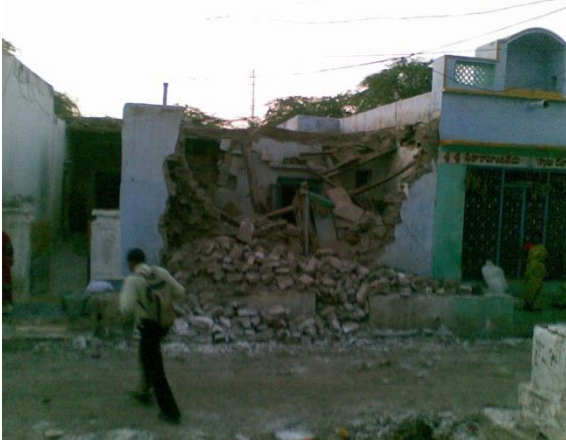
Photos 14 and 15: Collapsed buildings
