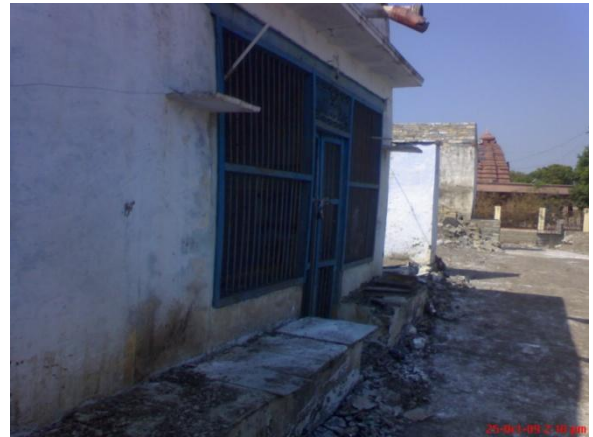
Photo12 : Locked houses even after a month
