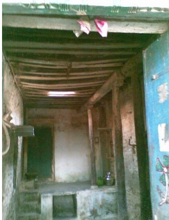
Photo 10 : CRS building in mud mortar
