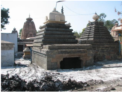
Photo 4: Silting around the temple
