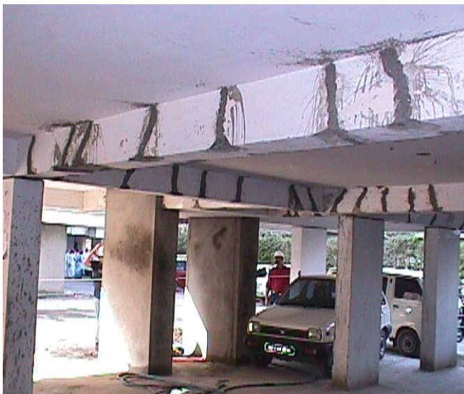
Photo-9: Spiral cracking in beams
