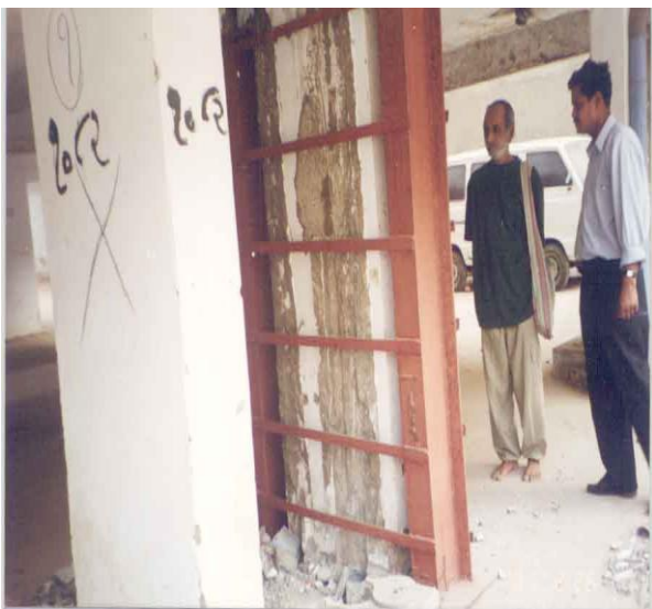
Photo-12: Improper retrofitting
