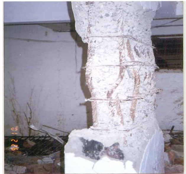
Photo-13: Poor detailing
