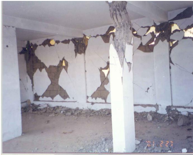
Photo-3: 'X' cracking in walls
