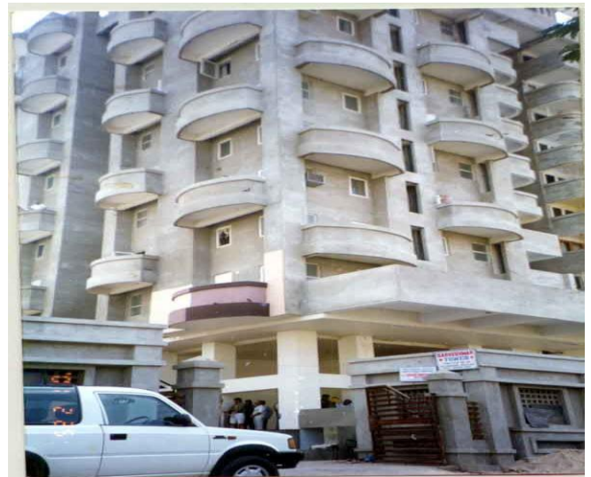
Photo-5: Floating columns
