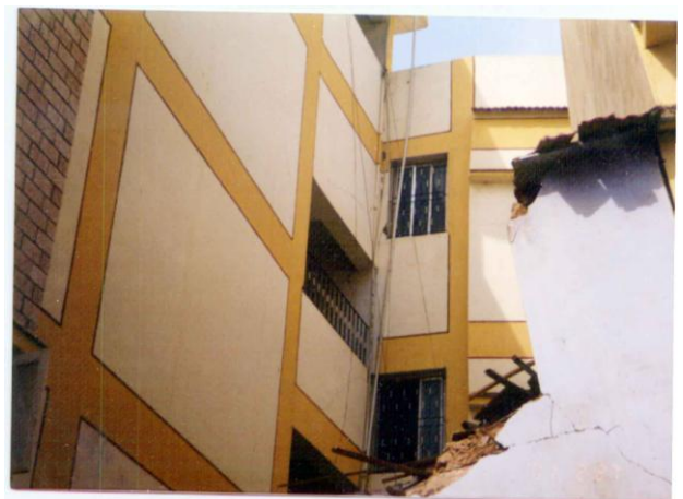
Photo-11: Pounding of buildings
