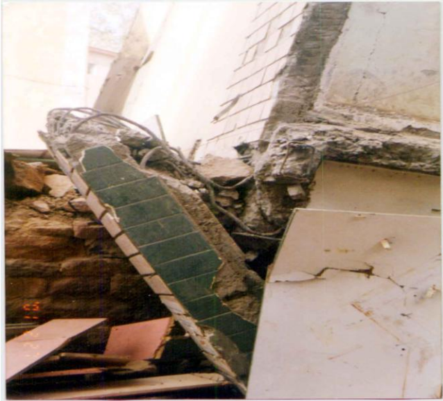
Photo-8: Fractured Columns
