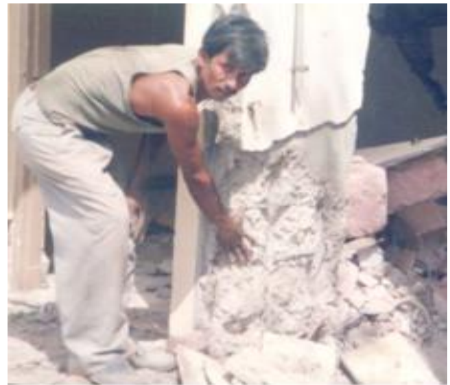
Photo-14: defective workmanship
