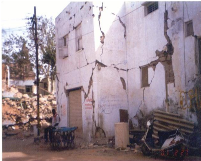
Photo-4: Wide spread cracking in building
