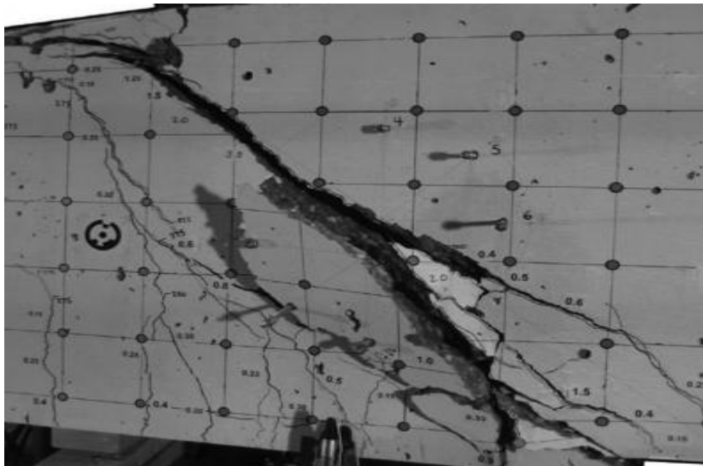
(c) Compression strut failure
