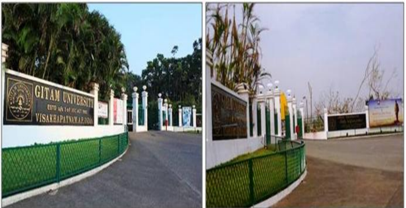
Fig 1 (a) View of Main entrance gate of Gitam University before and (b) after the cyclone.
