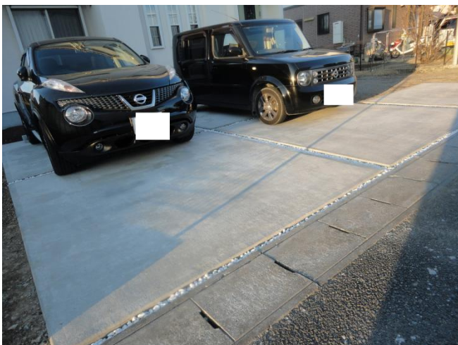
Fig. 6: Parking lot produced with Econ ® in Shizuoka area
