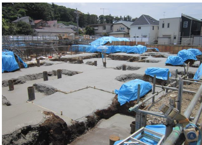
Fig.7: Concrete basement with Neomix ® in Yokohama area
