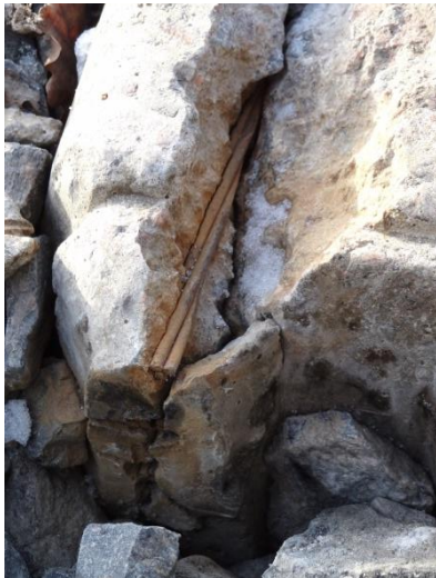
Fig. 6: The damaged sleeper front; [source the authors archive].
