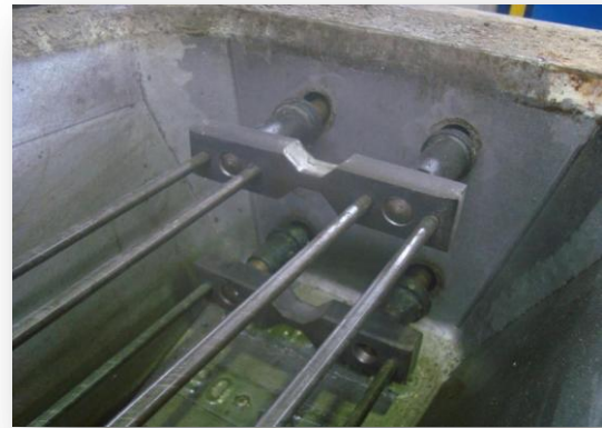
Fig. 8: The damaged sleeper front. Source the authors archive.
