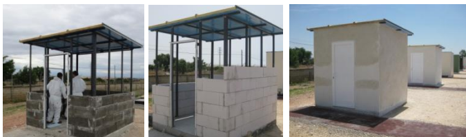
Fig 7 Mockups being built with GREEN CAST blocks (left) and Ytong ones (center). Both mockups finished (right).
