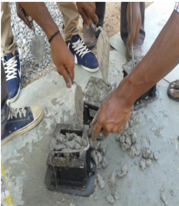
Fig-2: Placing of Geopolymer concrete
