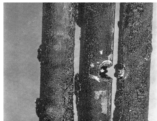
Fig -6: Spot arc damage to conductor caused by arcing through charred insulator [1]
