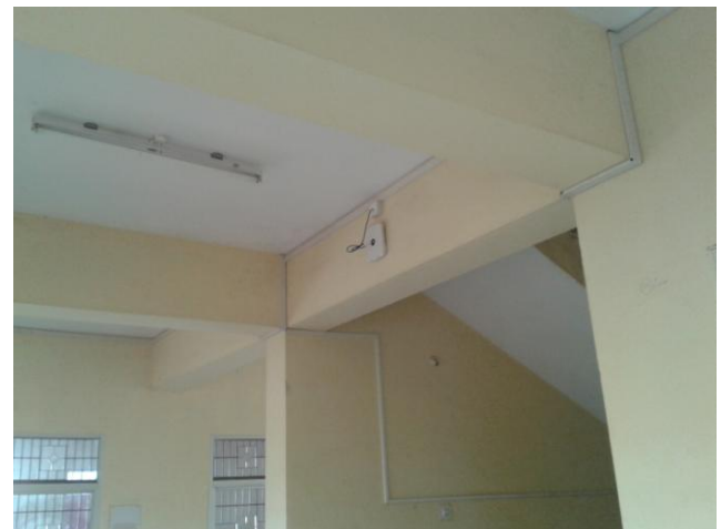
Fig: 1 Wi-Fi access point
