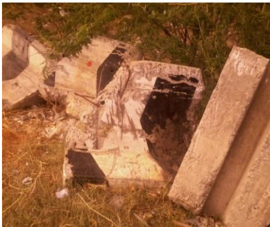
Fig -2.4: RCC Jersey Barriers
