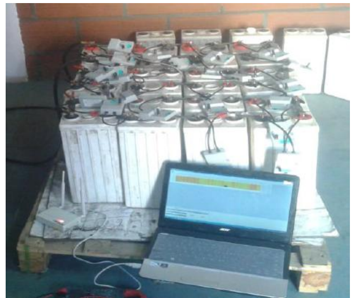
Fig -1: Experimental BMS setup picture.
