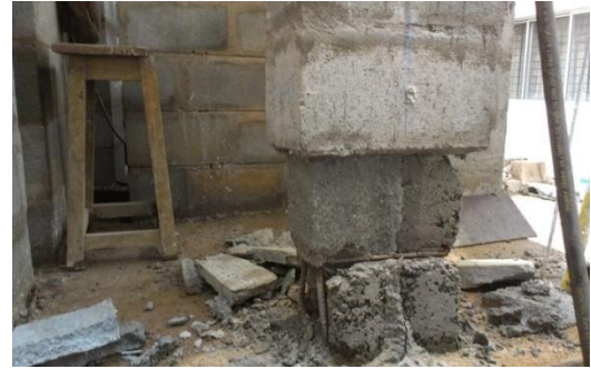
Fig 3(g) Spalling of block material
