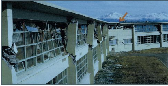
Fig-2: Damages Caused to the Roof Diaphragm at the Re-entrant Corner of West Anchorage High School, Alaska, during the 1964 earthquake
