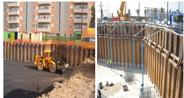
a. Cantilever method b. Tie back method
