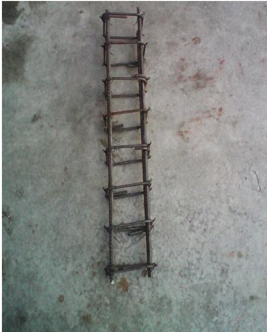
Fig -1: Cage of Beam
