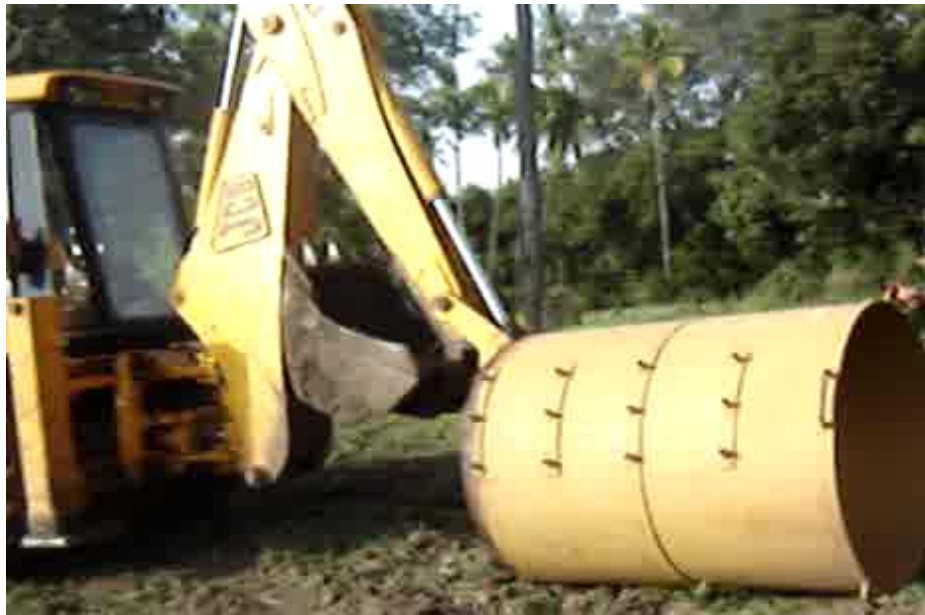
Fig -2: Lysimeter Installations
