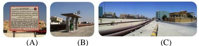
(A) Just instruction and warning board to prevent the pipe not the peoples (B) Bus stop is very close to the oil pipe, which cause dangers to the passengers (C) The oil pipe is installed in which no barriers or pavement to prevent the cars to crush the pipe, which might cause some accident with huge fire
