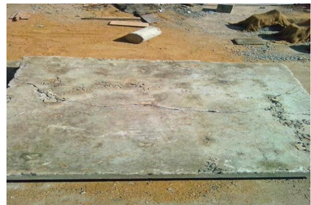
Fig: 2.1 Crack Pattern on slab after loading
