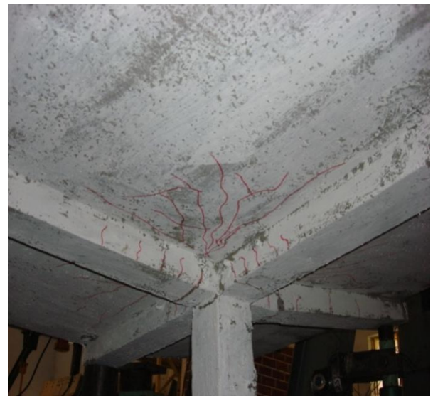
Fig. 22 Crack pattern of Beam-Column joint (BCJ) specimen
