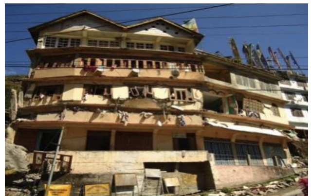
Fig 1: Collapse of one inter-mediate story in of the Moonlight School five-story RC frame building at Chungthang, Sikkim [16].
