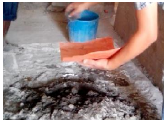
Fig-2: Mixing of steel fibers in mortar
