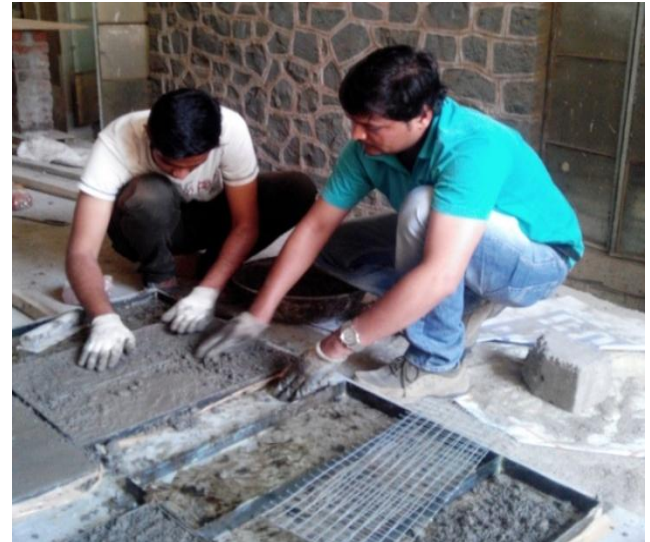
Fig-7: Placing of layers in mortar
