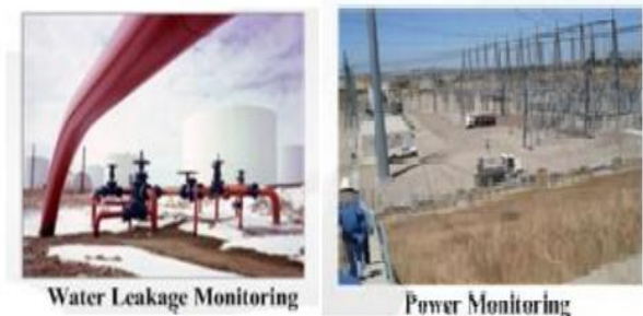
Fig 1: Water leakage Monitoring, Power Monitoring
