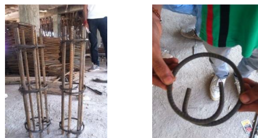
Fig1 (a) Steel Cage (b) 8mm Circular Steel Tie
