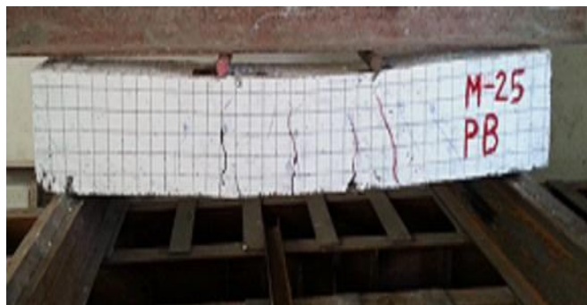
Fig -5: Crack pattern in Control Beam
