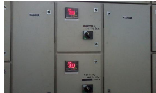
Fig -2: Panel of Energy Meter
