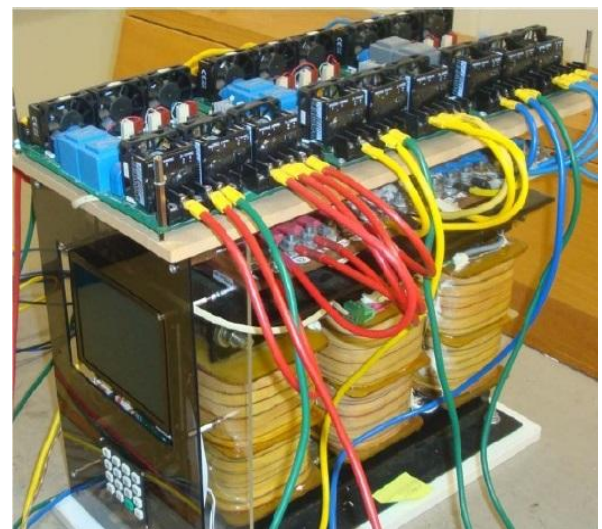
Fig-1: Three-Phase 10-kVA Switchable Transformer
