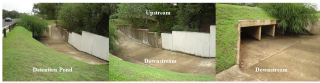
Figure 1a Detention Pond-Type 1 with stepped rectangular weir for flow control (Courtesy: City of Austin, TX)
