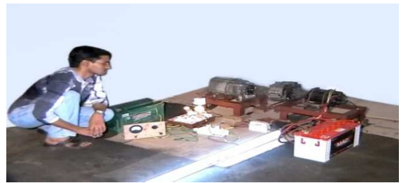
Fig 6:- ON Position Generator
