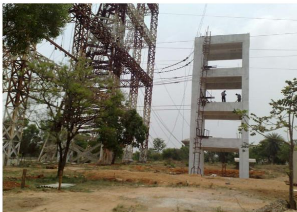
Fig- 16: Tower Testing Facility at CPRI, Bangalore
