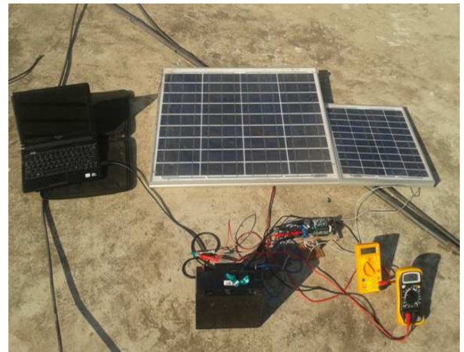
Fig -17: Complete installation of MPPT tracker
