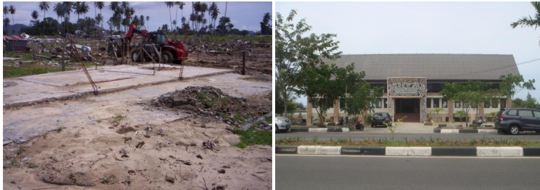
(a) (b) Fig – 3: Condition of building after the tsunami (a) building damaged by the tsunami, and (b) new building
