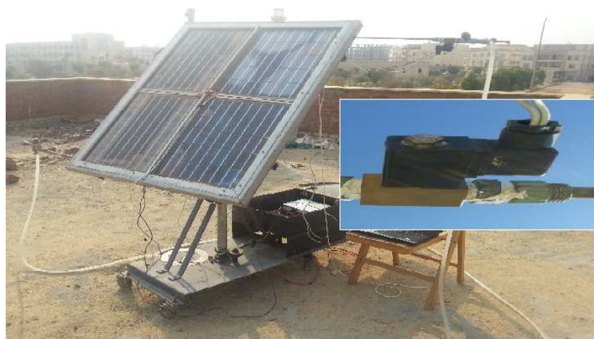
Fig (6): Place of electrical valve used to decrease the temperature of PV surface modules.
