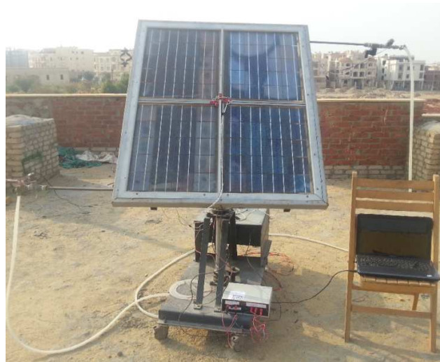
Fig (7): General view of the experimental system used.
